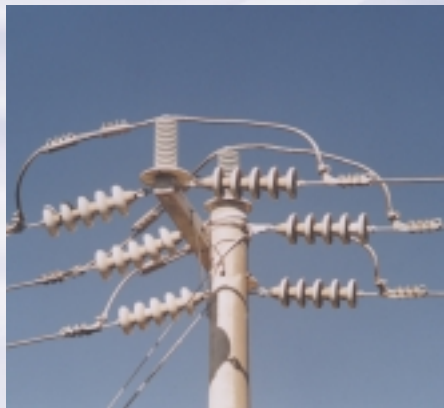
Disc and line post insulators used on overhead lines
